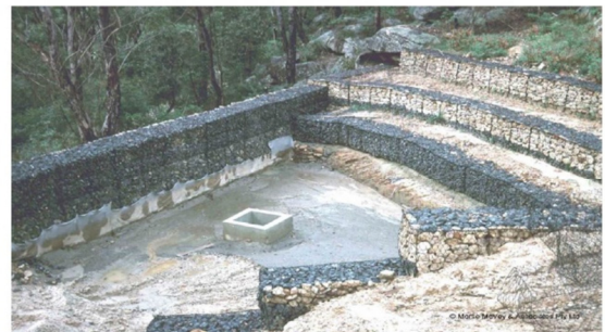
Photograph 6-3 Type C gabion sediment basin on steep terrain, later converted to a permanent facility.
