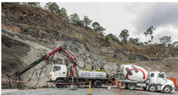
Shotcreting completed by Jemna and Holcim
