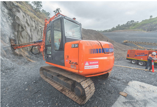
Rock Bolting completed by Team Rock Anchors and Bluey
