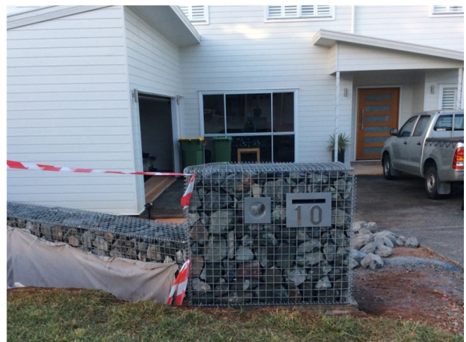
Letterbox and Retaining Wall in Final Stage of Construction
