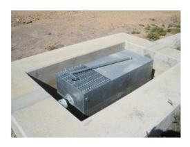
In the event of a major spill/emergency, the ball valve can be closed between the third chamber and the storm water outlet, thus eliminating external contamination.
